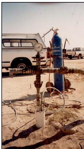
Fig-3: Pressure Grouting Set-up for a site in Al-Hufoof.
