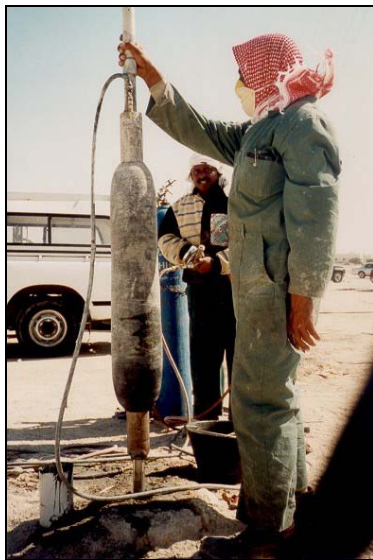
Fig-2: Inflatable Packer for Pressure grouting.
