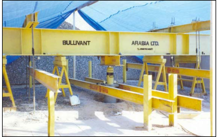
Pile Test Arrangement on Site
