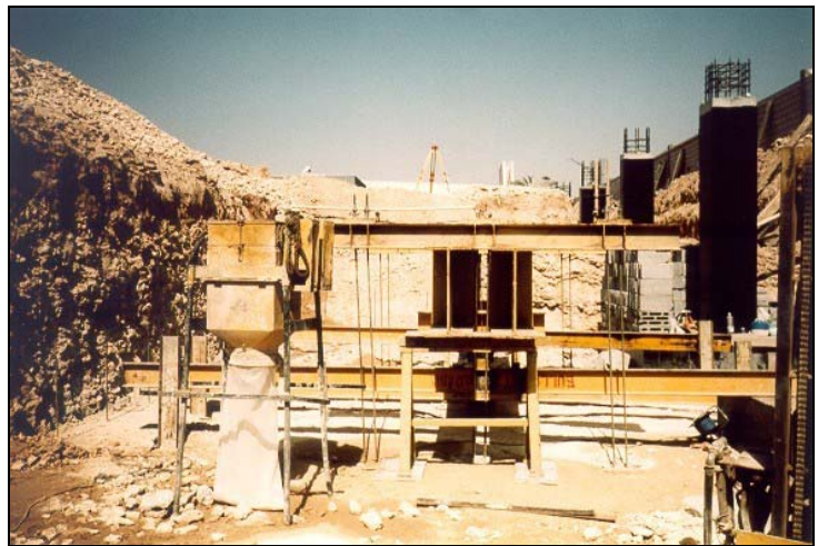
Pile Testing Sectional View on Site
