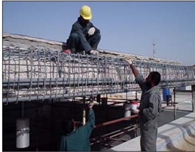
Repair of Beam damaged by corrosion of Reinforcement
