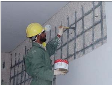
Patch Repair of Concrete wall damaged by corrosion.
