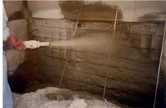
Reinstatement of corroded wall
