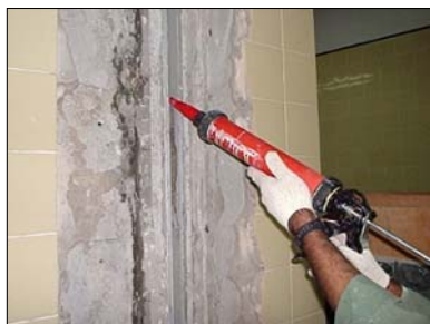
Repair of Expansion Joints
