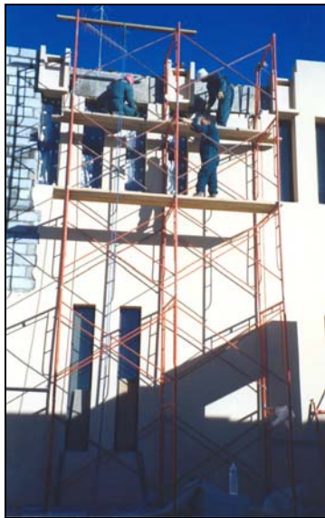
Repair works in King Khalid Stadium, Tabuk
