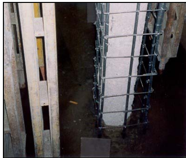
Reinstatement of Column
