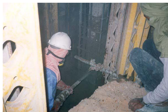
Reinstatement of Column
