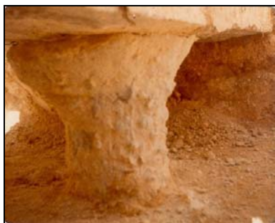
Fig-7: Shape of Minipile below Isolated Footing
