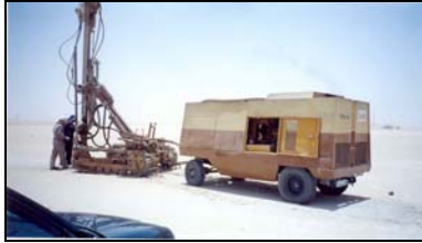
Fig-4: Track Mounted Rig & Compressor
